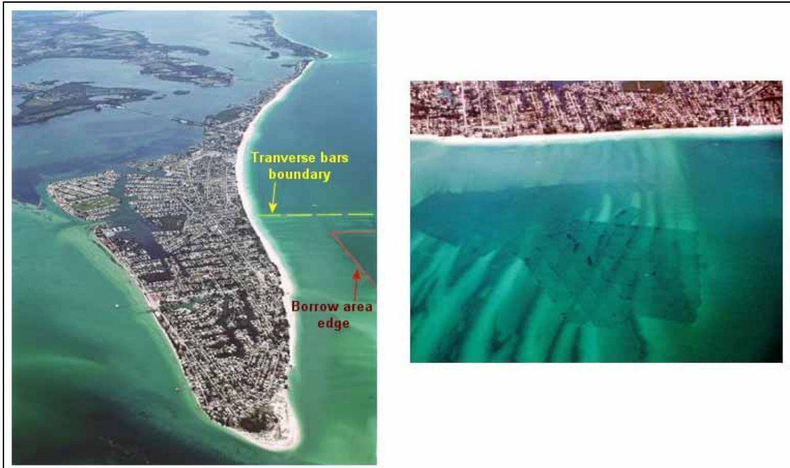
Figure 10. North-south oblique aerial photograph (left image) showing the drumstick shape of Anna Maria Island. The landward boundary of the 2002 borrow area (arrow marking the borrow area edge) is located within the transverse bar field. The transverse bars and the 2002 borrows, shown in the right image (looking from west to east), abruptly terminate to the south in a relatively featureless nearshore.
